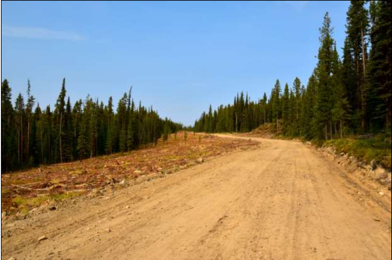
Figure 3 - A portion of the Gibbons Pass Road 8-mile long clearcut.
