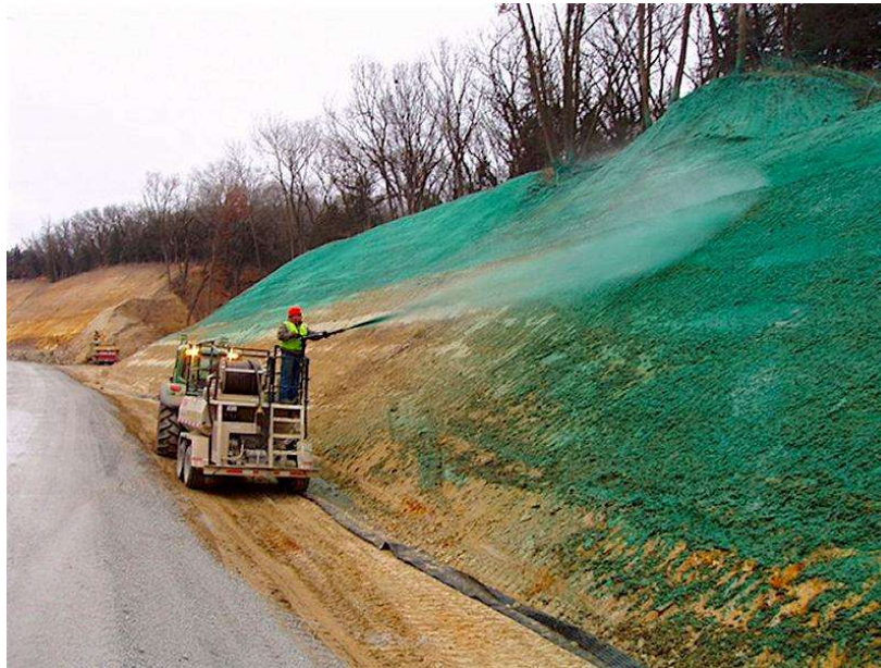
Hydroseeding for Erosion Control
