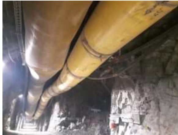
Vent Bag in a Development Heading (area)
