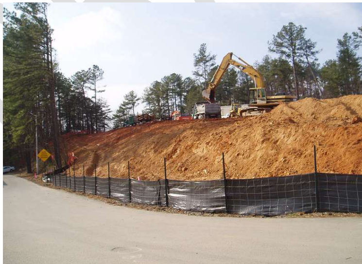
Silt Fence for Erosion Control
