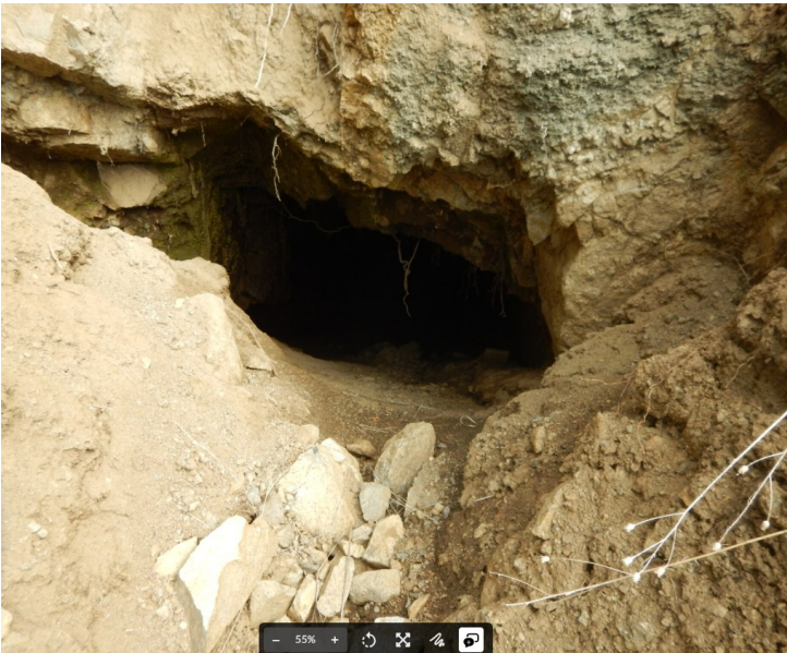
Above Image 2: Open adit #1, Approximately 2ft high, 3 ft wide opening, dry.
