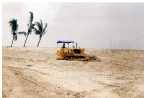
FIG. 15. Backfilled mined out area.
