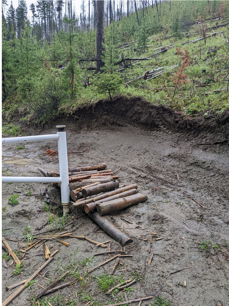
Figure 12: Breach created for wider motorized vehicles that are illegal past the gate.
